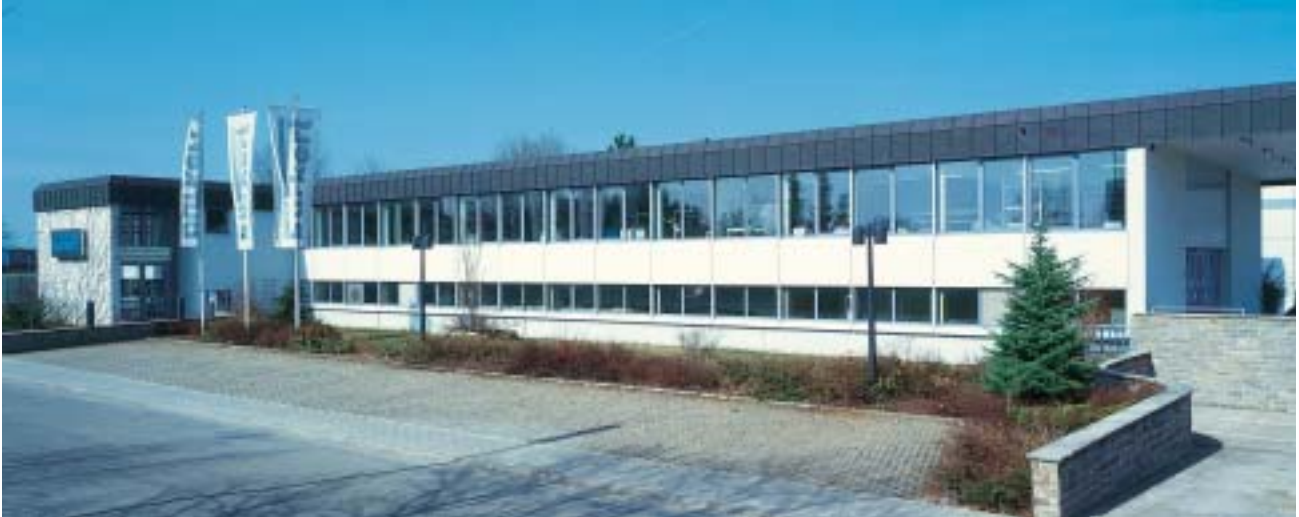
MicroFluidics production facility in Gerabronn, Germany
